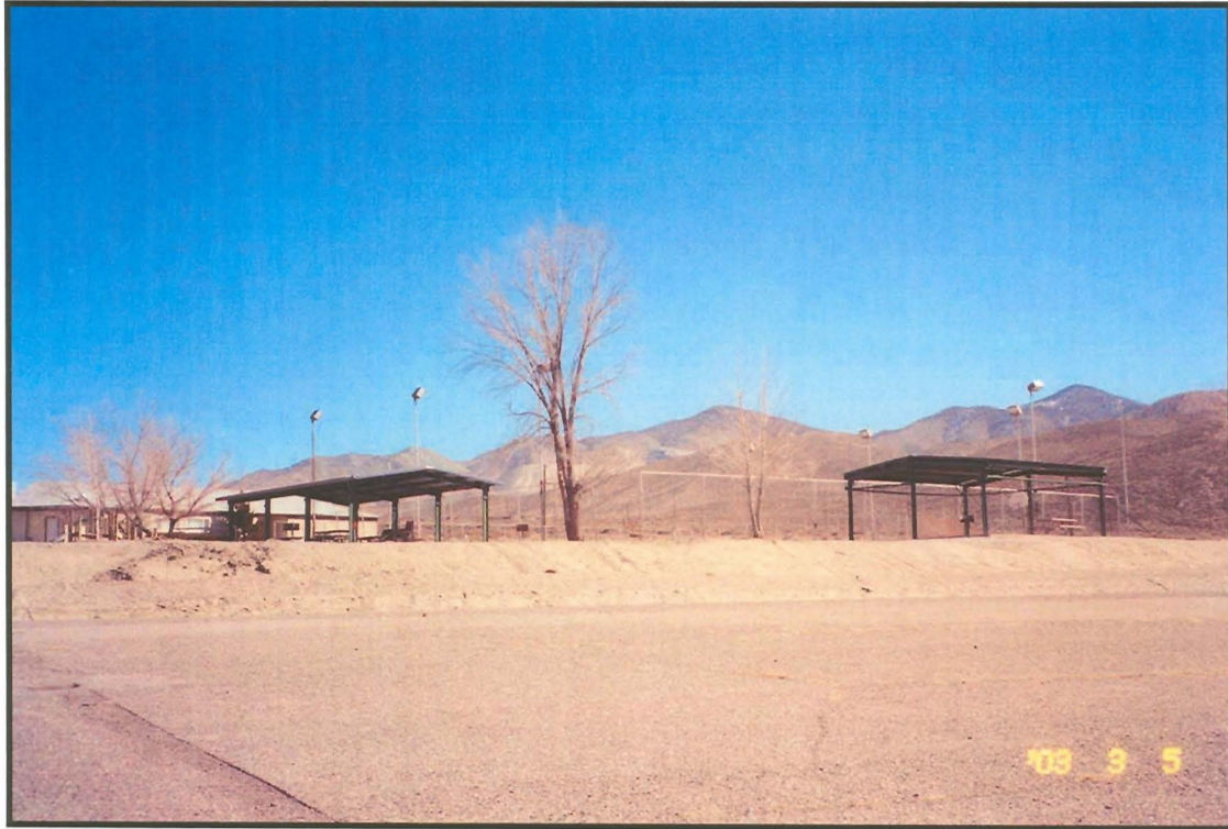
Photograph 6: View of park northeast of the subject site across "E" Avenue.
