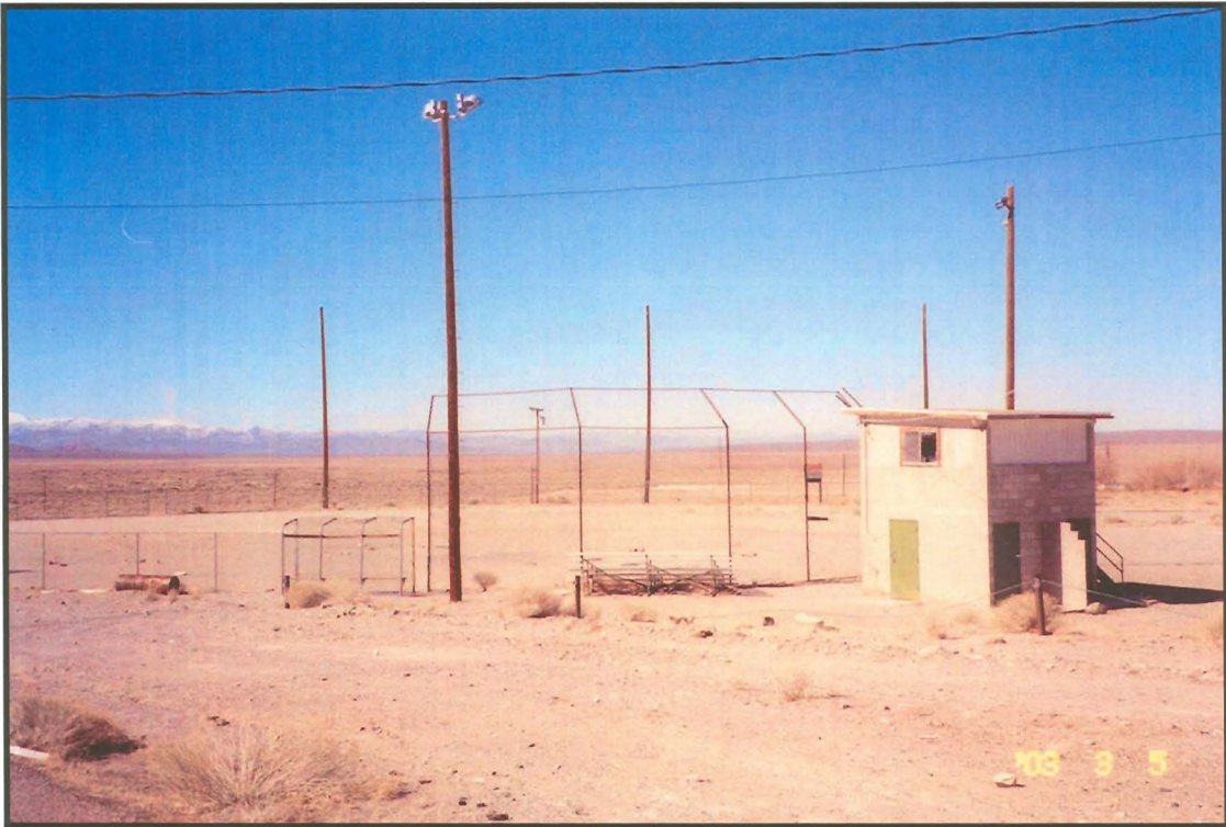
Photograph 5: View of baseball field on the west side of the subject building.
