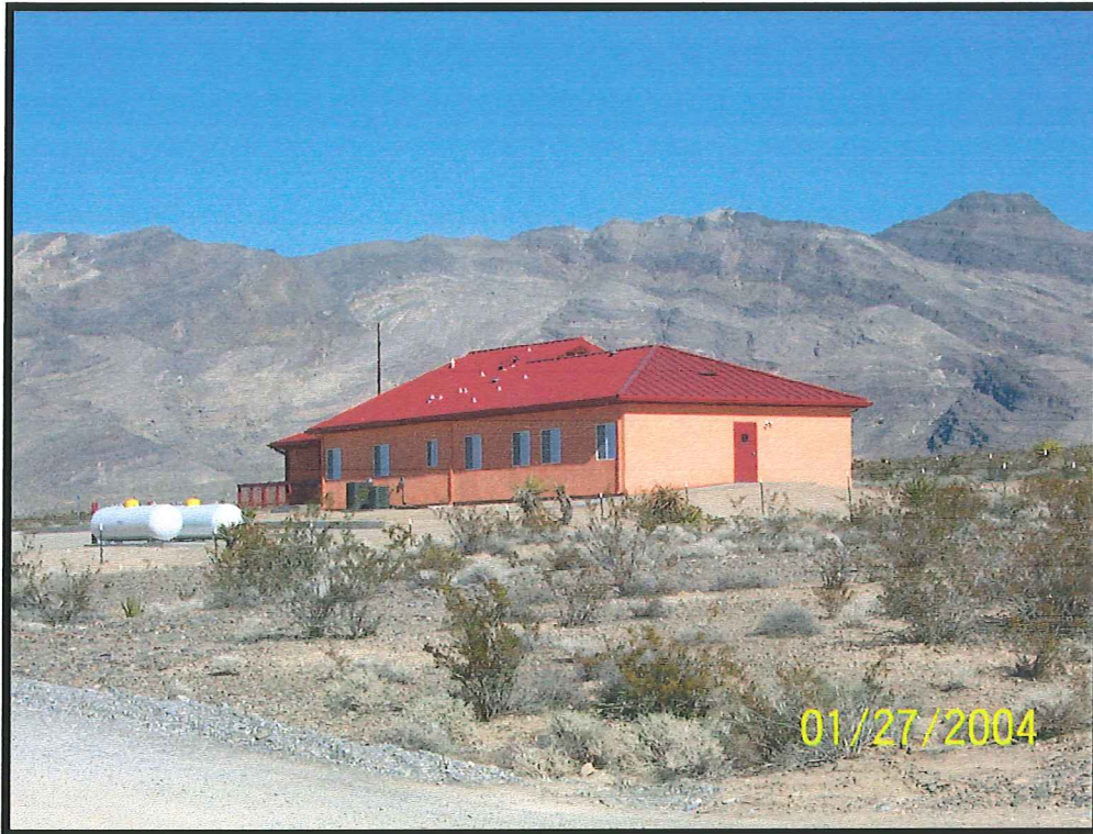
Photograph 7: View to the north of unoccupied BLM Fire Station.
