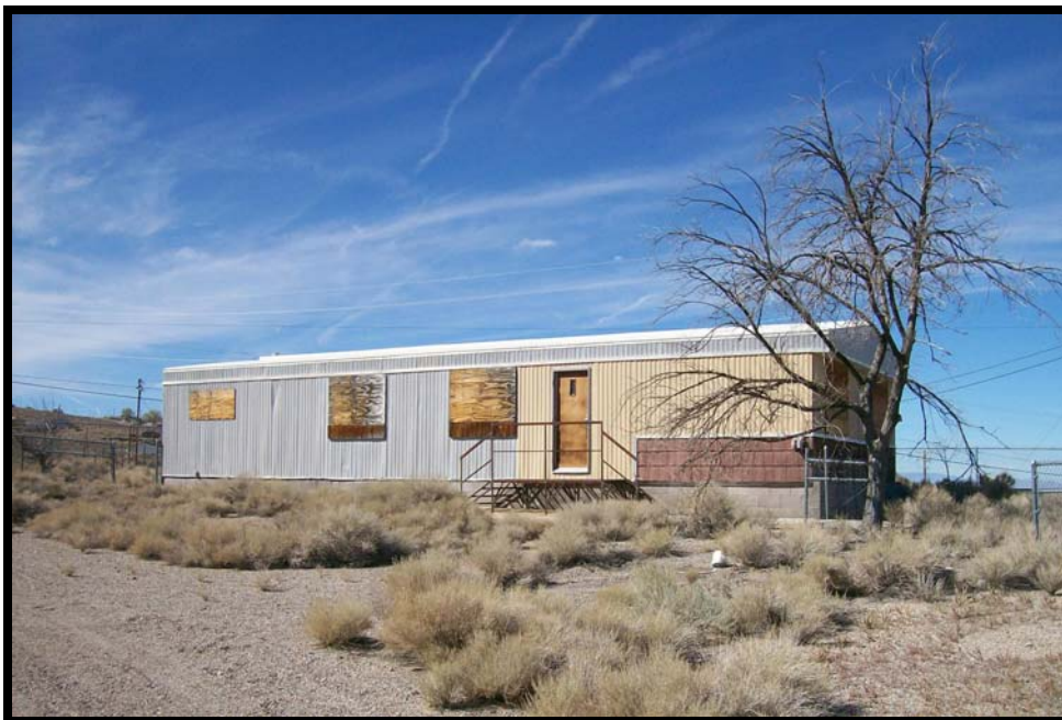
Photograph 4: View of unoccupied mobile home, facing northwest.
