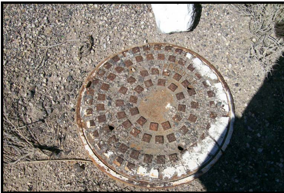
Photograph 12: View of sewer manhole cover on subject site.
