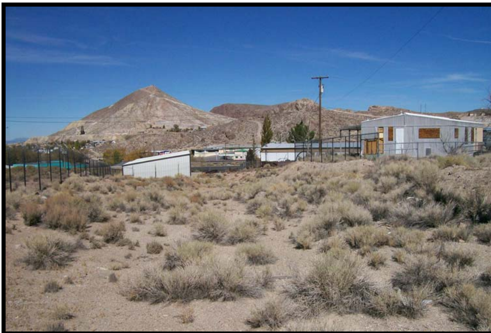
Photograph 10: View of drainage ditch on western margin of subject site, facing north.
