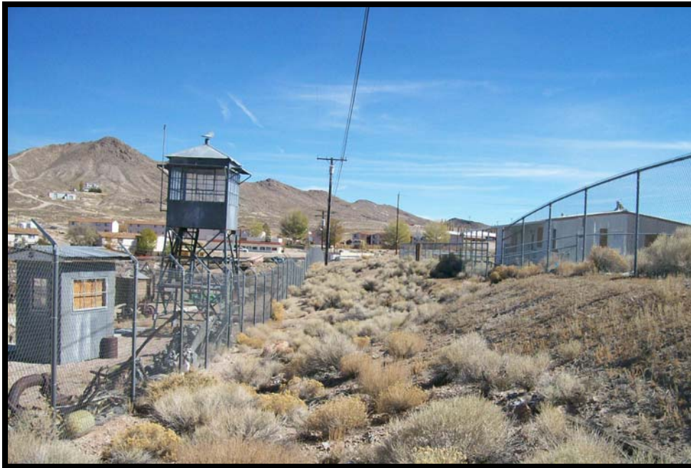
Photograph 11: View of drainage ditch on northern margin of subject site, facing east.
