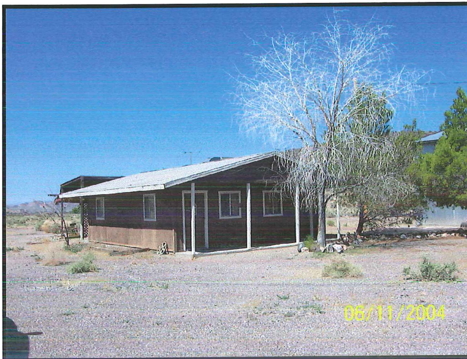
Photograph 18: View of mine office building on Section 28 Township 11 South, facing southwest.
