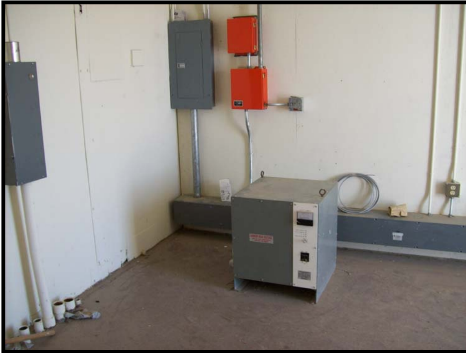
Photograph 13: View of unused electrical equipment inside airport office building.
