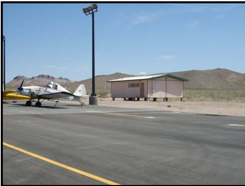
Photograph 6: View of wooden building on northeast corner of airplane parking area, facing northeast.
