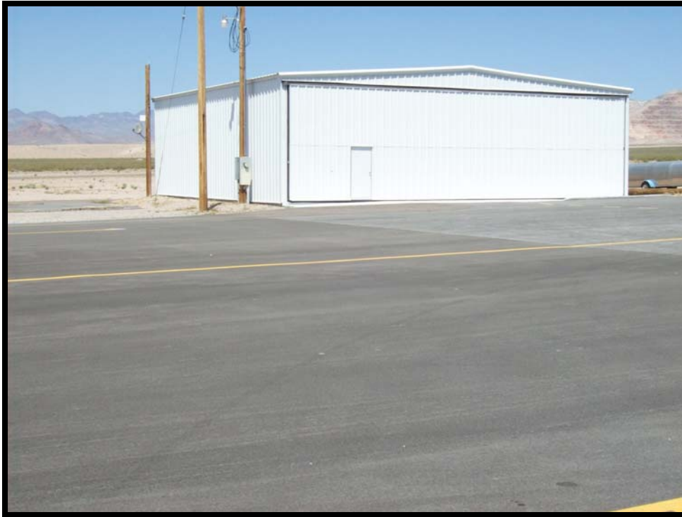
Photograph 3: View of metal county-owned building, facing northwest.
