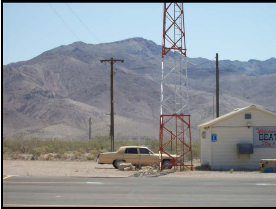
Photograph 1: View of airport office building, facing northeast.
