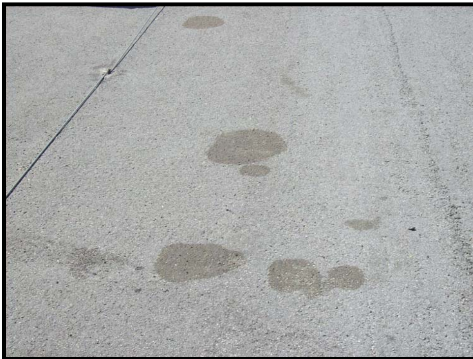
Photograph 8: View of pavement staining associated with trailer-mounted fuel storage tank owned by Great Basin Soaring.
