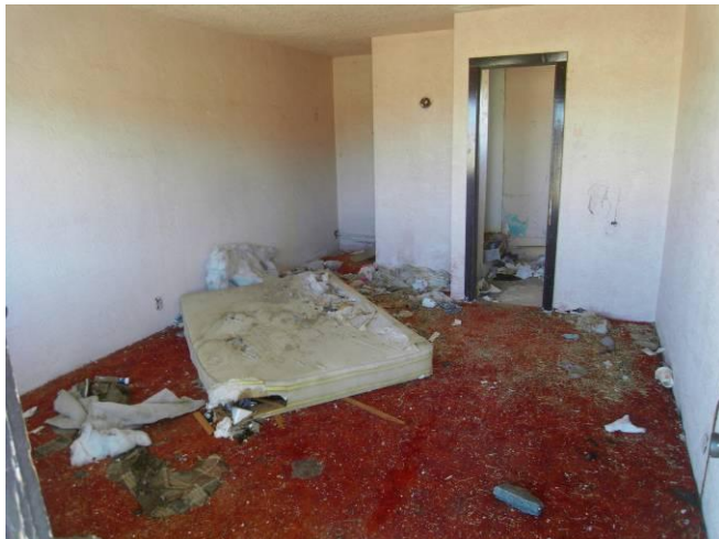
Picture 21. Interior view of a typical motel unit.
