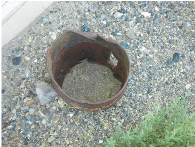
Picture 25. Another steel casing of unknown use (possibly septic) behind motel unit.
