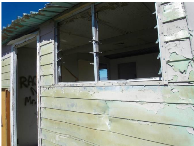
Picture 23. Exterior view of a typical motel unit (note multiple layers of peeling paint).
