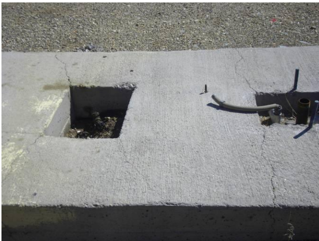
Picture 43. Additional view of former pump island.
