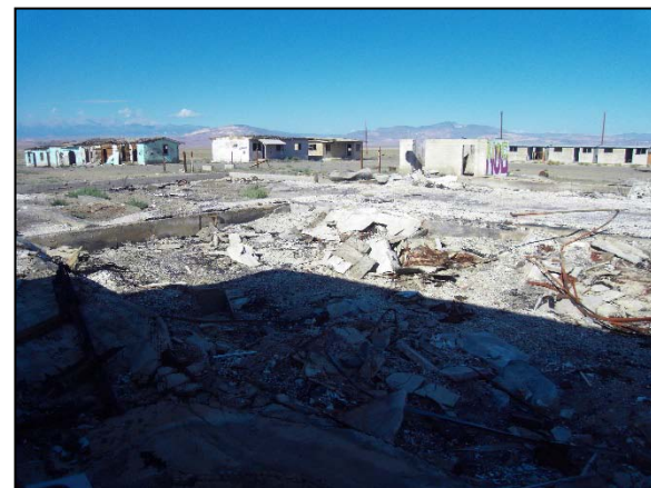
Photograph 24: View of Burned Structure (looking southwest).
