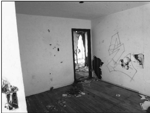
Photograph 19: Interior view of Building 8, Motel Units (looking southeast).
