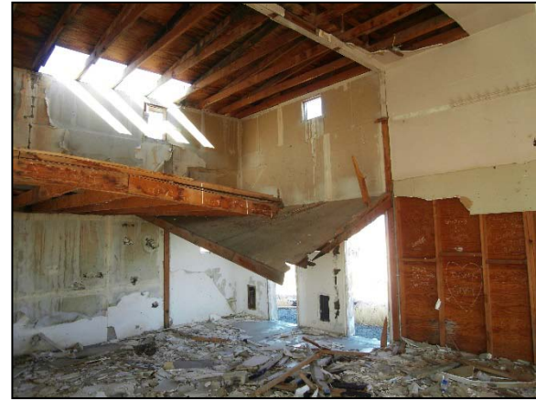
Photograph 2: Interior view of Building 1, former Service Garage (looking west).
