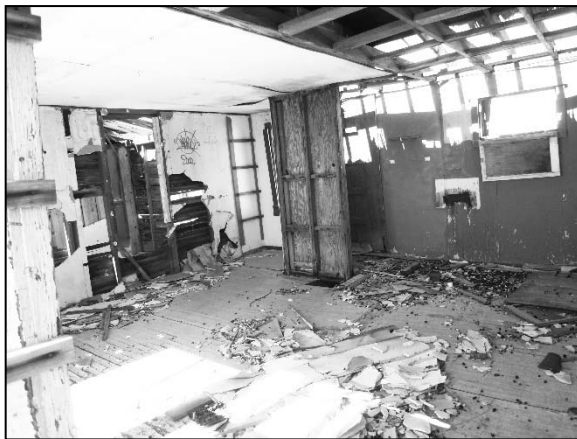
Photograph 23: Interior view of motel unit in Building 10, Motel Units (looking southwest)
