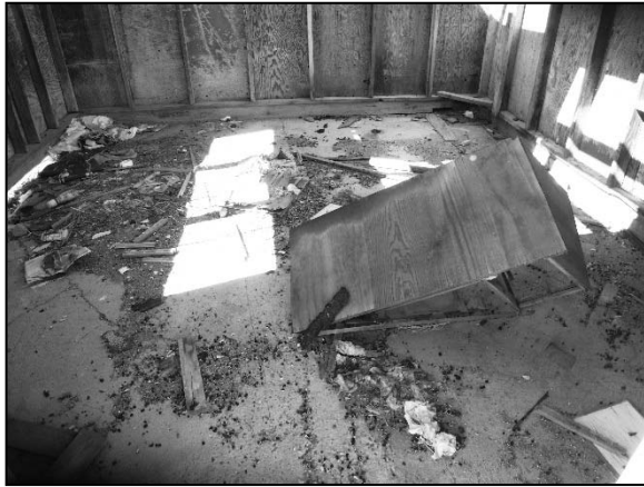
Photograph 5: Interior view of Building 2, Former Hydraulic Tank House (looking south).
