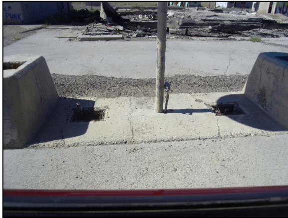
Photograph 25: View of Gas Dispenser Island (looking southwest).
