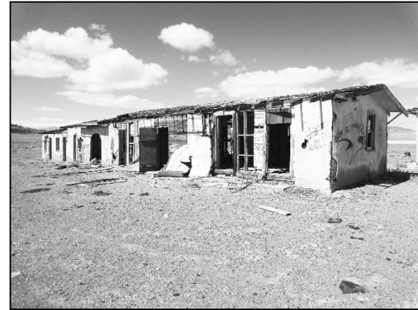
Photograph 22: Exterior view of Building 10, Motel Units (looking southwest).
