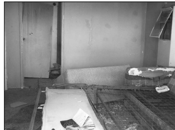
Photograph 16: Interior view of motel unit in Building 7, Motel Units (looking northwest).
