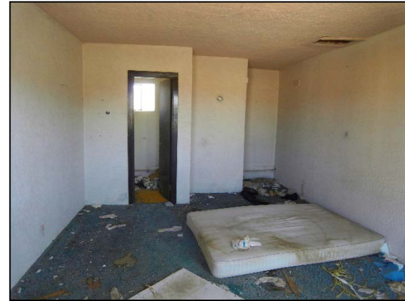
Photograph 14: Interior view of motel unit in Building 6, Motel Units (looking northeast).
