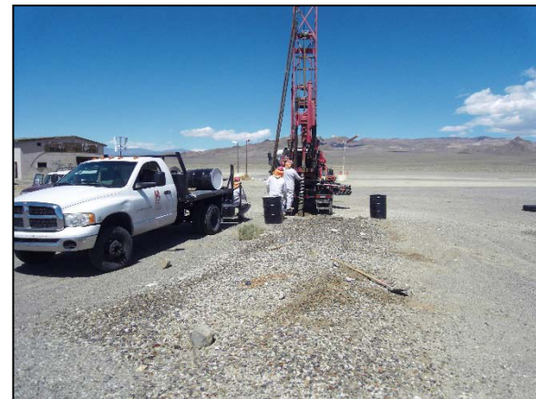
Photograph 28: Boring SB-3 (looking north).
