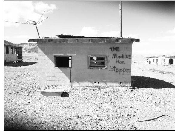
Photograph 6: Exterior view of Building 3, Diesel Generator House (looking southwest).
