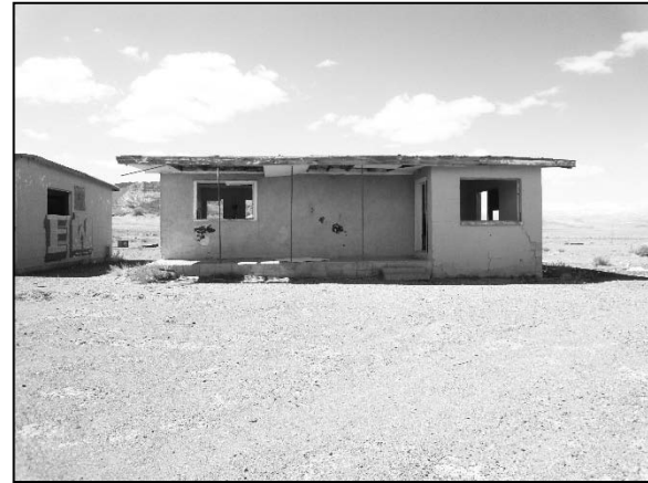
Photograph 18: Exterior view of Building 8, Motel Units (looking southwest).
