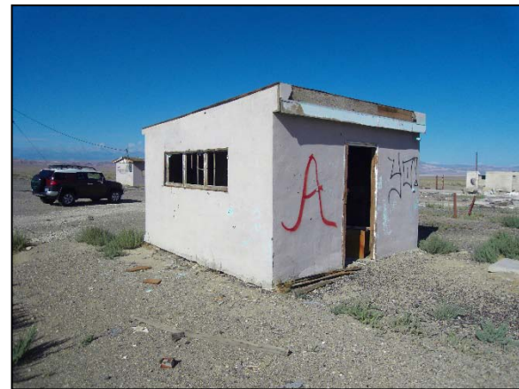
Photograph 4: Exterior view of Building 2, Former Hydraulic Tank House (looking southwest).
