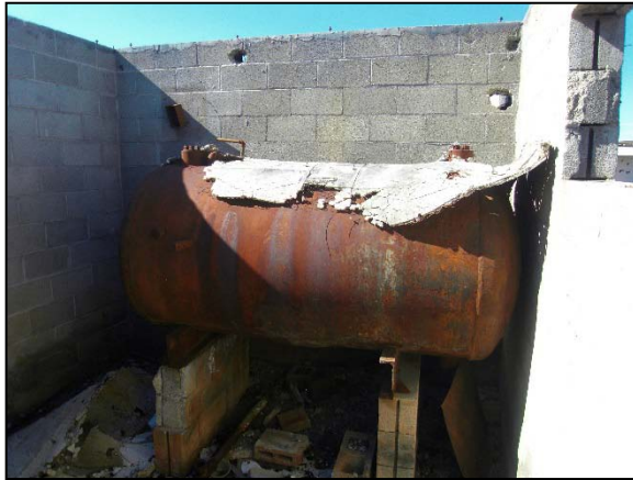
Photograph 9: Interior view of Building 4, Shower House (looking southwest).
