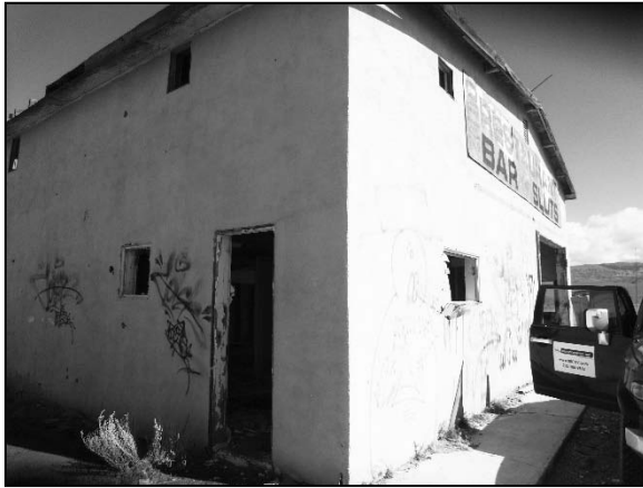
Photograph 1: Exterior view of Building 1, former Service Garage (looking north).
