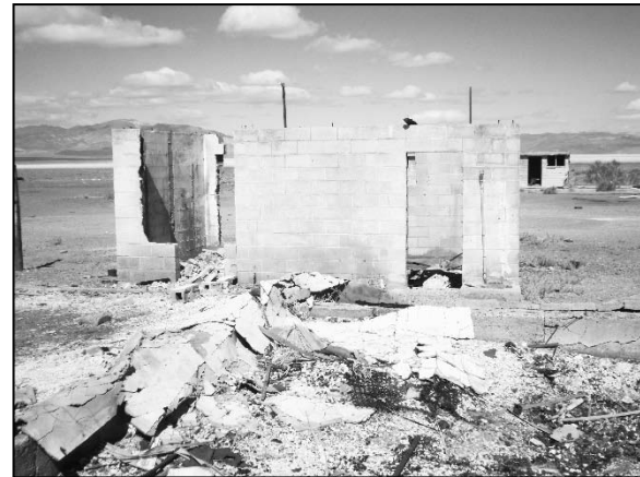
Photograph 8: Exterior view of Building 4, Shower House (looking west)
