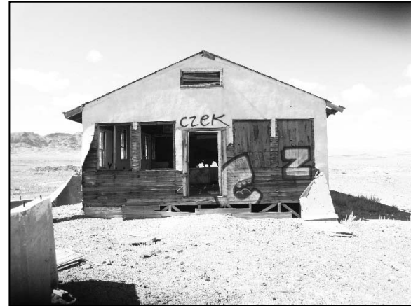
Photograph 10: Exterior view of Building 5, Motel Unit (looking southwest)
