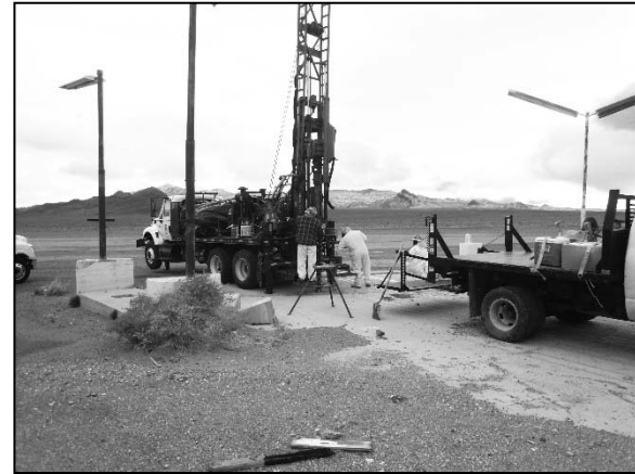
Photograph 30: Boring SB-5 (looking north).
