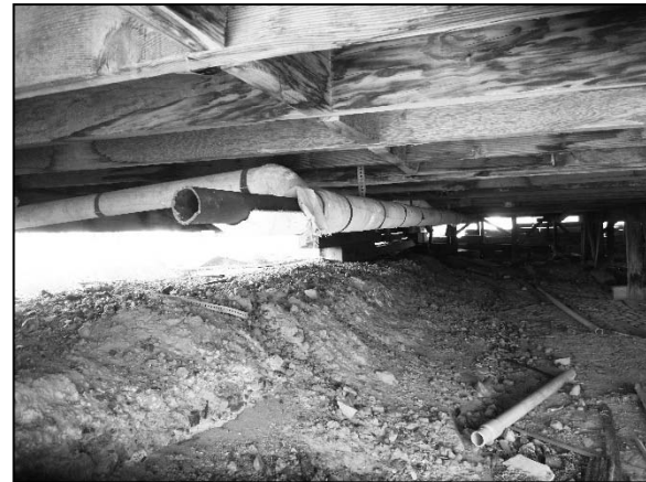
Photograph 12: Thermal system insulation below Building 5, Motel Unit (looking north).
