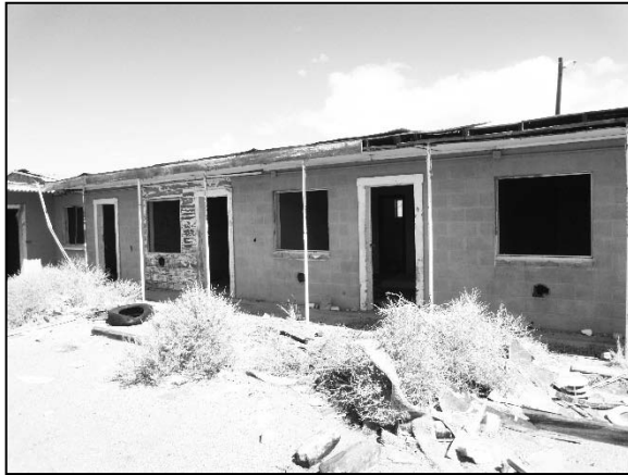
Photograph 13: Exterior view of Building 6, Motel Units (looking north).
