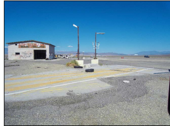
Photograph 26: View of the west Diesel Dispenser Island (looking west).
