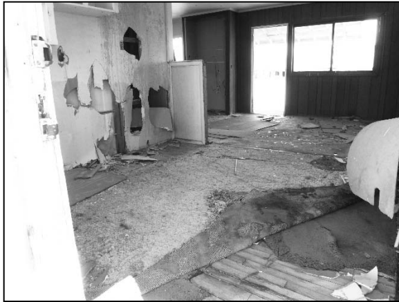
Photograph 21: Interior view of Building 9, Motel Units (looking north).
