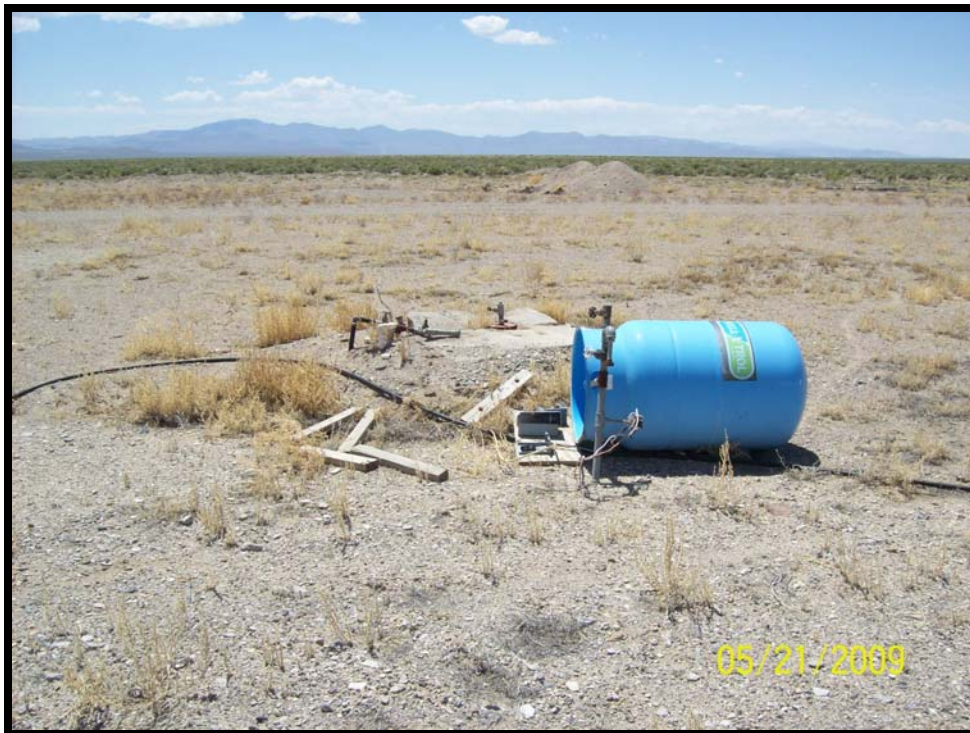
Photograph 11: View of abandoned water supply well and settling tank west of hangar, facing west.
