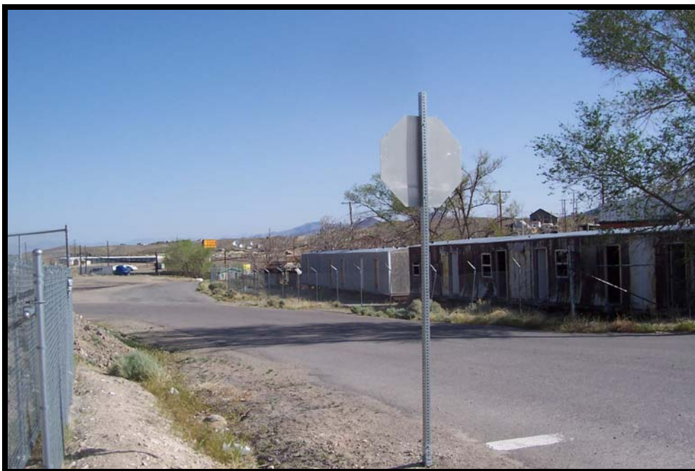
Photograph 4: View of west margin of site along Summit Street, facing north.
