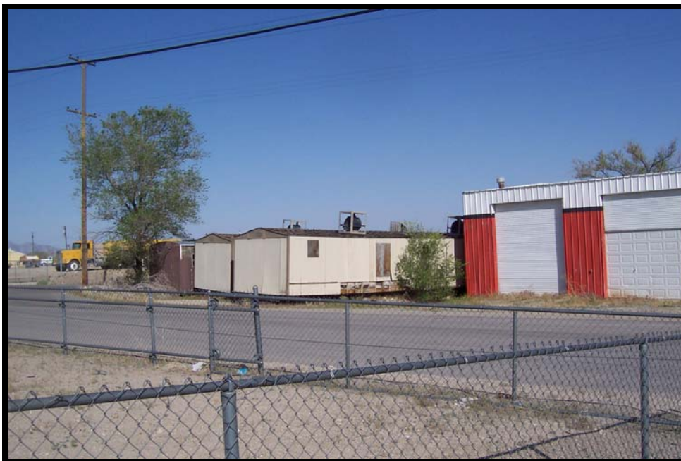
Photograph 2: View of trailers on west side of subject parcel 08-061-05, facing northwest across Knapp Avenue.
