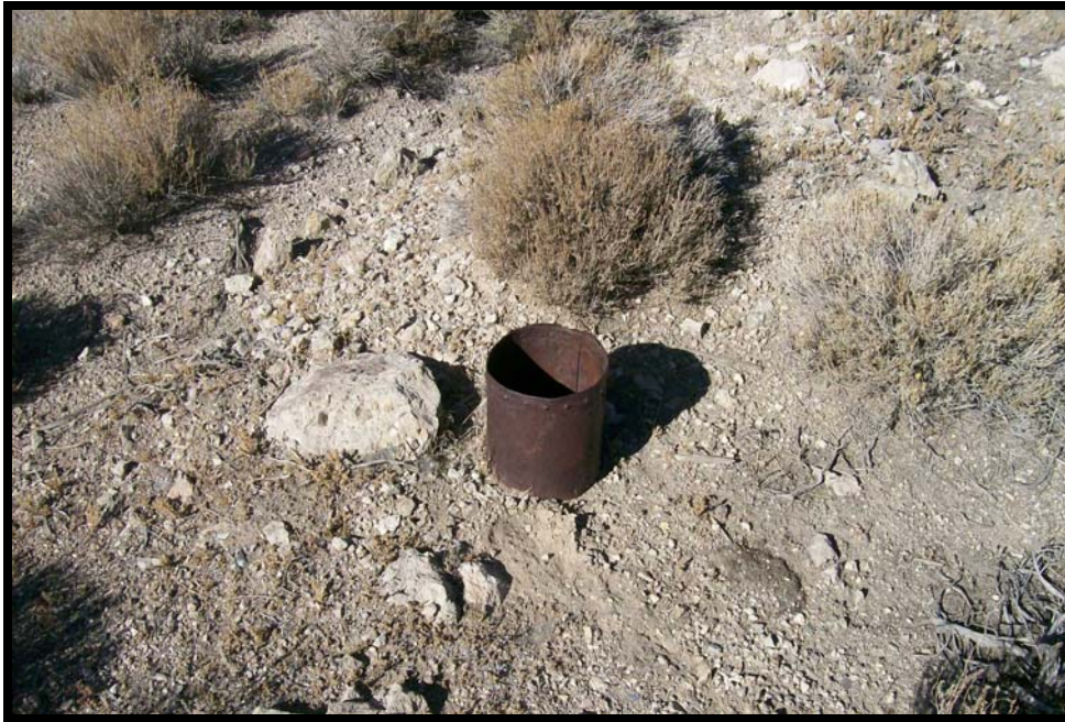
Photograph 9: View of possible water valve associated with concrete foundation pad.
