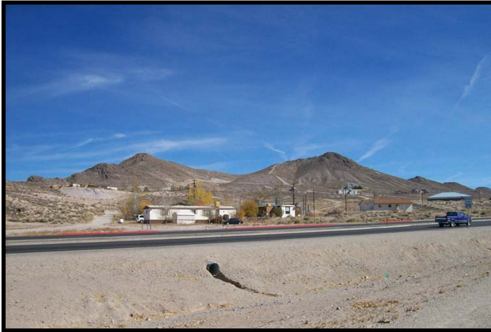
Photograph 3: View of southeastern adjoining residential properties, facing east across U.S. Highway 95.
