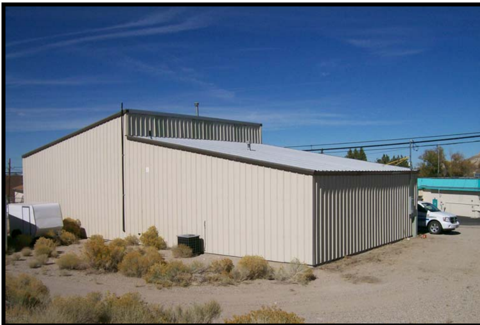
Photograph 12: View of Nye County Emergency Services ambulance bay near western margin of subject site, facing northwest.
