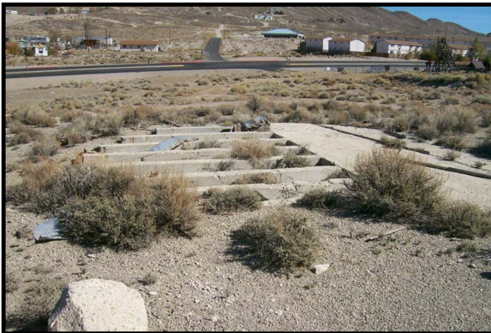
Photograph 8: View of concrete foundation pad near center of subject site, facing north.
