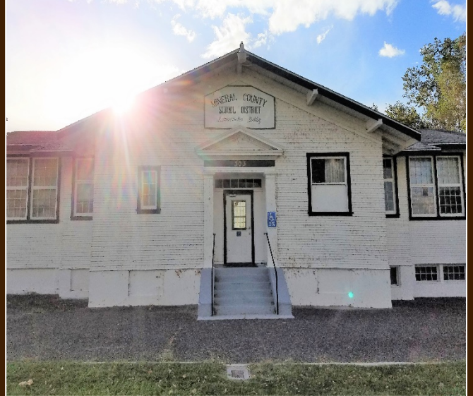
MCS D Administration Building Photo
