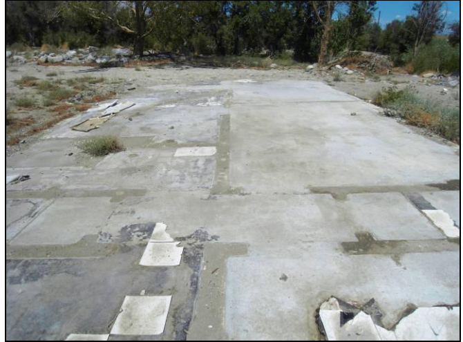
Photograph 45. Settling pond located adjacent to the east side of the concrete "racetracks". Water exiting the fish hatchery operation was first passed through this settling pond prior to being discharged back to Oak Creek.
