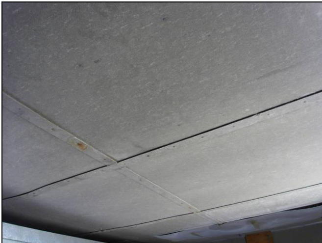
Photograph 11. Transite panel ceiling material in freezer room.
