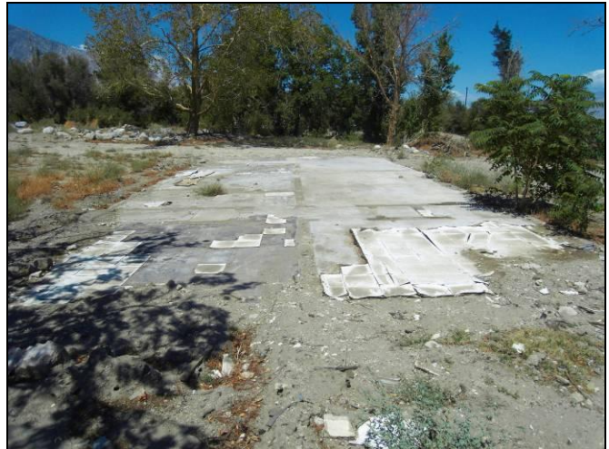
Photograph 47. Close up view of the vinyl tile/mastic on the foundation from Photograph 46.
