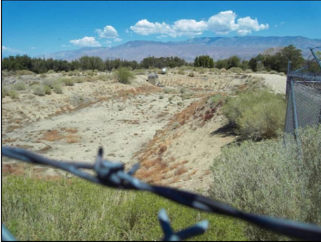
Photograph 45. Settling pond located adjacent to the east side of the concrete "racetracks". Water exiting the fish hatchery operation was first passed through this settling pond prior to being discharged back to Oak Creek.
