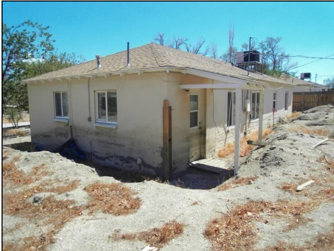
Photograph 49. Residential unit damaged during the flood event (note the waterline on the building walls).
