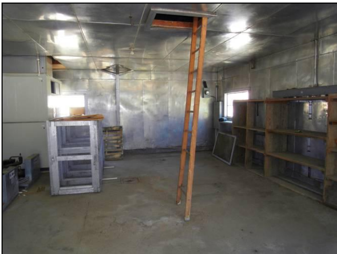
Photograph 7. Interior view of cold storage and feed preparation room.
