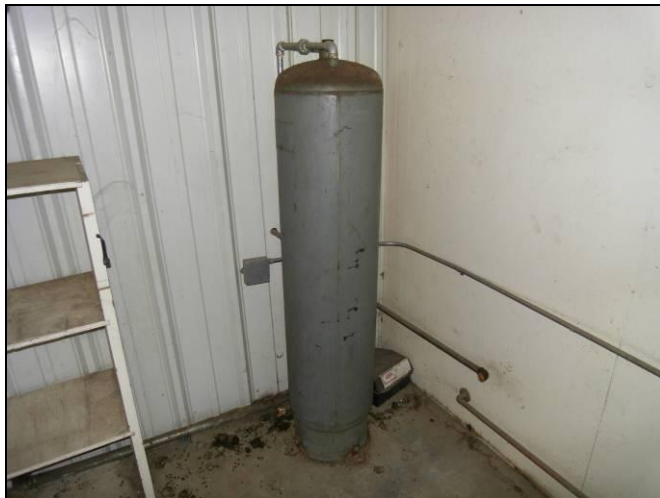
Photograph 29. Compressor tank located in the middle bay used for the hydraulic lift.
