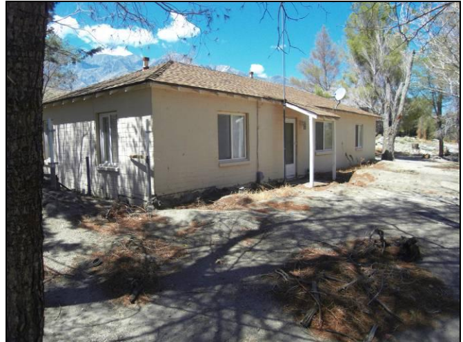
Photograph 49. Residential unit damaged during the flood event (note the waterline on the building walls).
