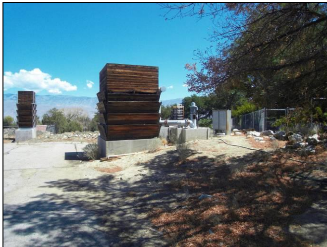
Photograph 44. View of the water treatment towers used to remove high concentrations of naturally occurring nitrates in the groundwater. The towers also serve the purpose of oxygenating the oxygen deficient water.
