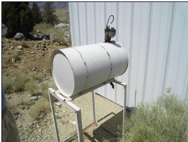
Photograph 31. Approximate 20-gallon drum tank (partially full) of an unknown petroleum product.
