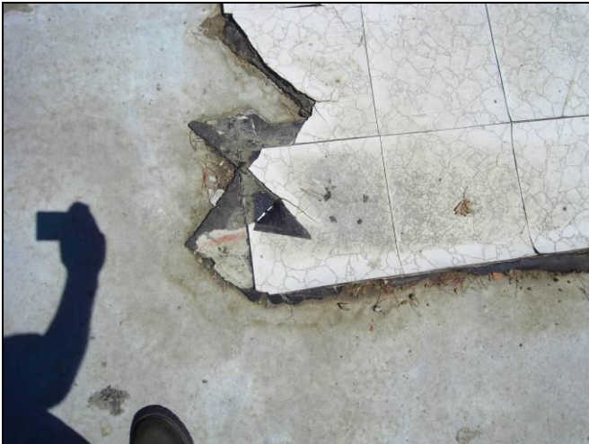
Photograph 47. Close up view of the vinyl tile/mastic on the foundation from Photograph 46.
