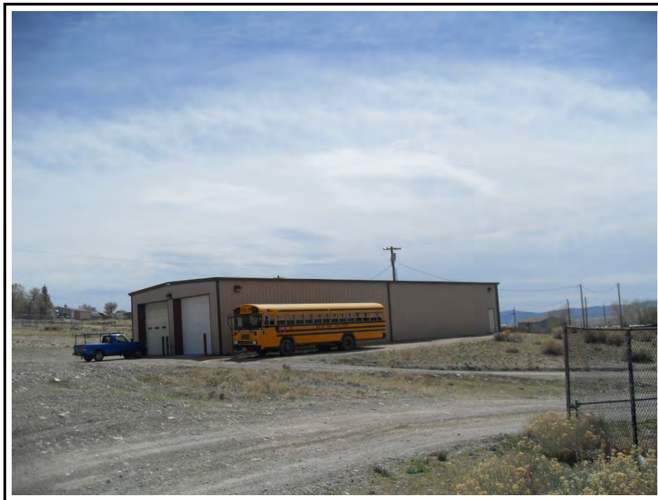
Photograph 7: Adjacent property to the south – school maintenance building
