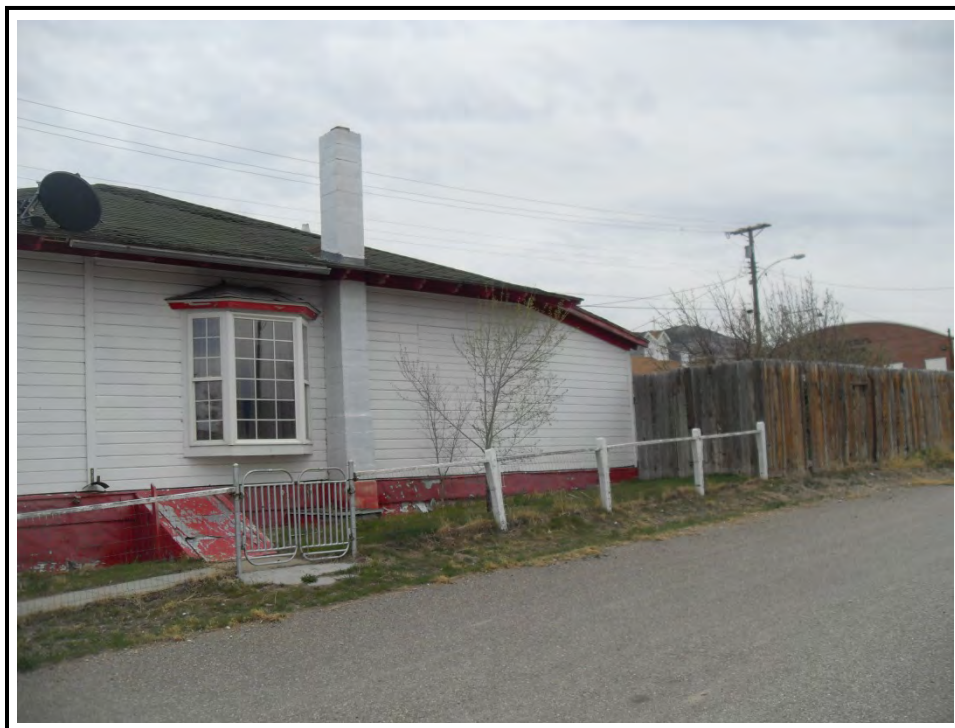
Photograph 8: Adjacent property to the east – residential
