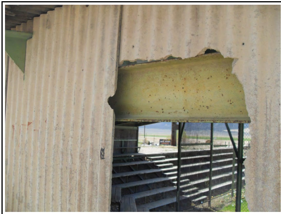
Photograph 17: View of siding – main field
