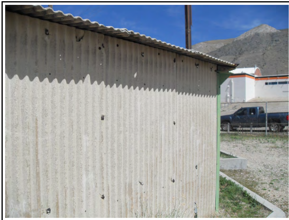
Photograph 21: View of siding and roofing – main field bleachers
