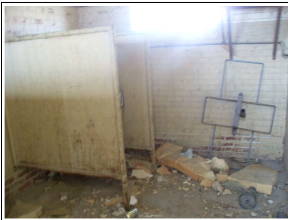
Photograph 30: View of bathroom interior
