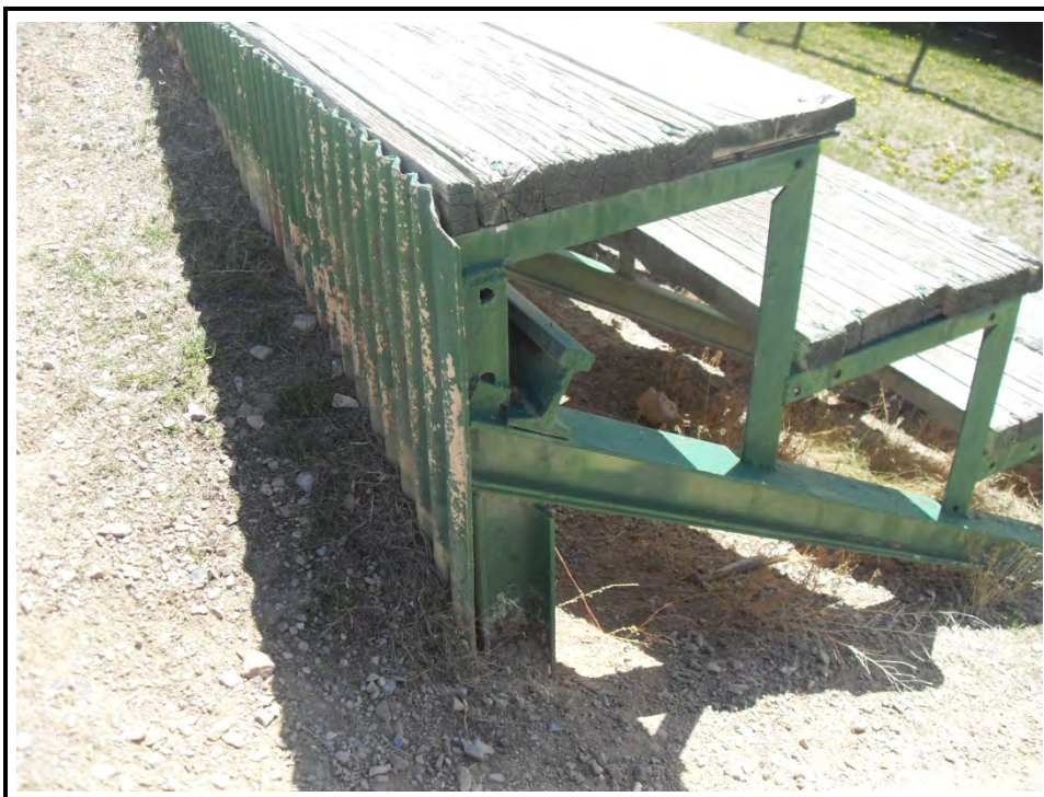
Photograph 20: View of typical siding and green paint on bleachers
