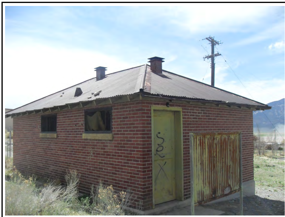
Photograph 28: View of bathroom structure of SEC
