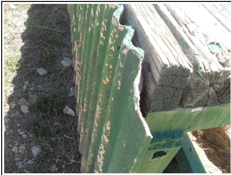
Photograph 23: Close-up view of siding - bleachers
