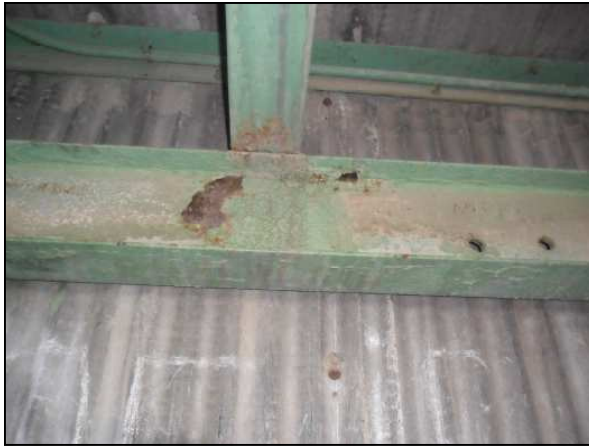
Picture 1 - Green Metal Beam Inside Grandstand.
