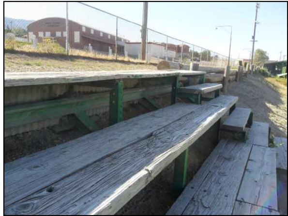
Picture 4 - Corrugated Transite Siding Behind the Outfield Bleachers. (From Below)
