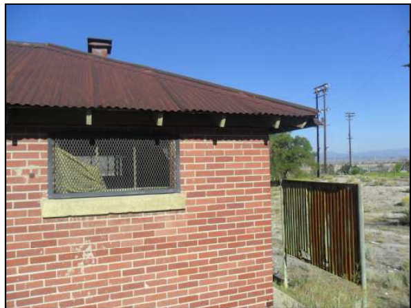
Picture 6 - Exterior Window Frame, Joists and Privacy Wall on the Restroom Building.
