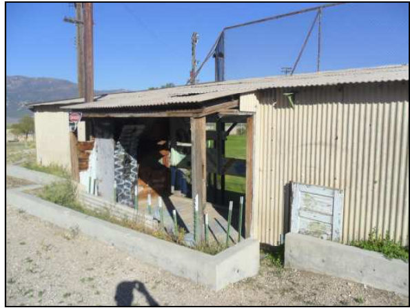
Picture 2 - Exterior Corrugated Transite Walls and Roof on the Grandstand.
