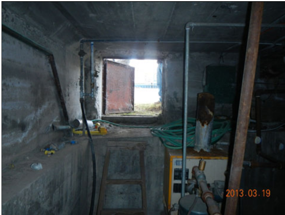
View of exterior access door from basement
