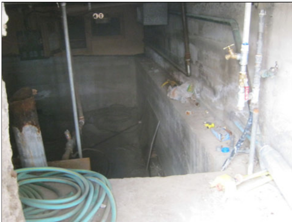
View of the basement area from the exterior door
