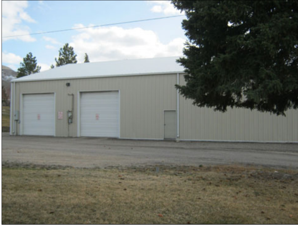
Adjacent property to the south – Fire and Ambulance Truck Garage
