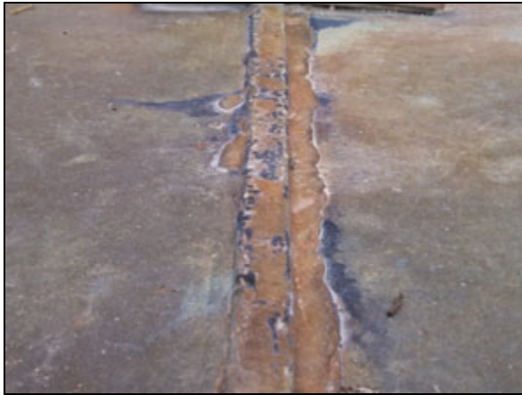
Picture 9—Leaded solder on the seam of the entrance roof.
