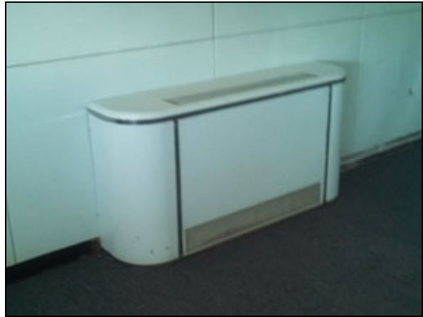
Picture 10—Lead paint on the blue metal radiator in the main room.
