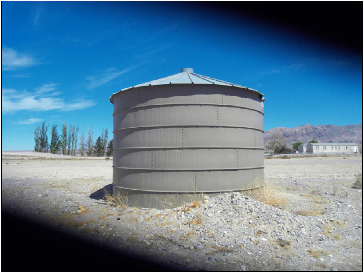
Picture 15. View on-site corrugated metal storage silo.
