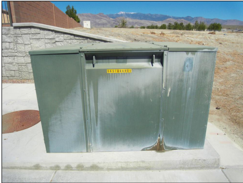
Picture 20. View of pad mounted transformer with minor leakage (approximately ¼ mile west of the subject site in the Mountain Falls residential community).
