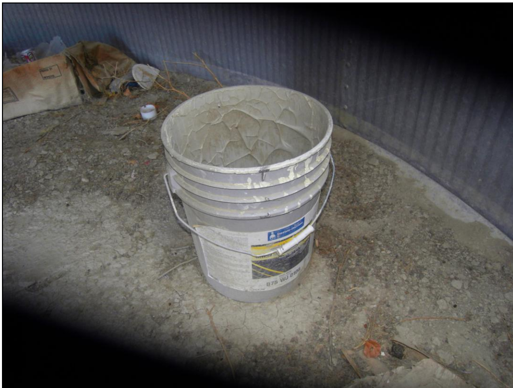
Picture 17. Interior view of corrugated metal storage silo with paint bucket.
