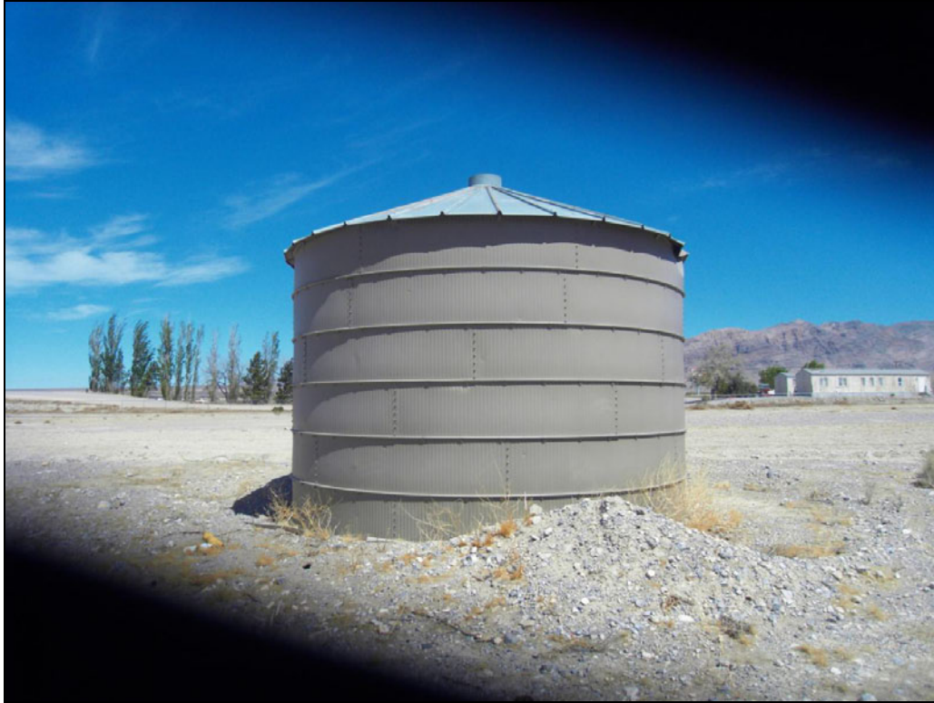
Picture 16. View on-site corrugated metal storage silo.
