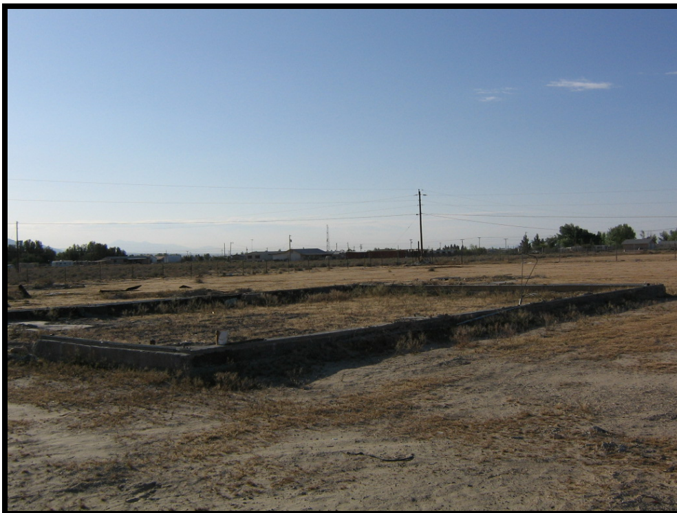
Photograph 2: View of perimeter foundation near eastern margin of site, facing southeast.
