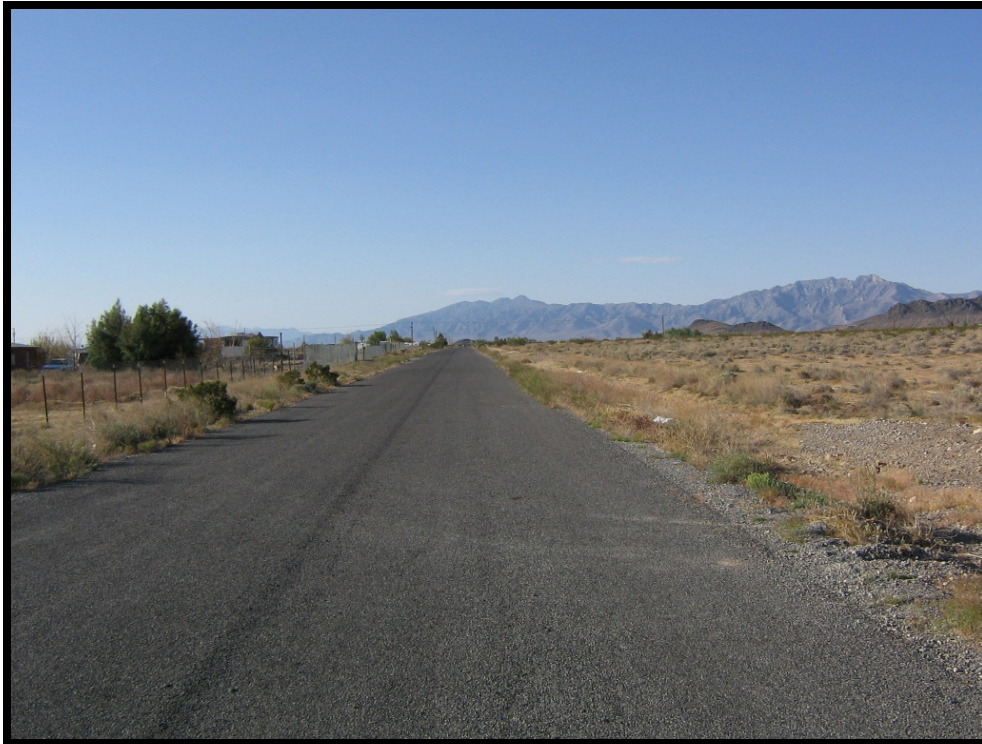
Photograph 11: View along Stephanie Street, facing south.
