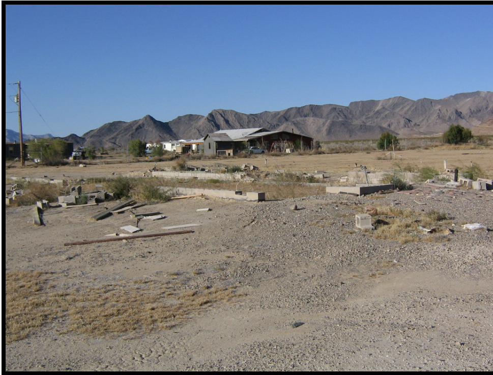
Photograph 3: View of perimeter foundation near center of site, facing southwest.
