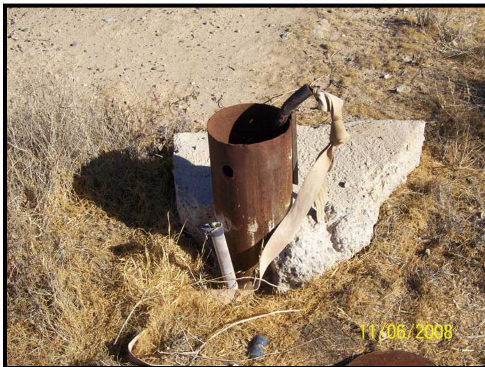
Photograph 6: View of site water well with open casing.
