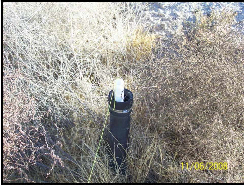
Photograph 7: View of disposable bailer placed in vent pipe associated with septic system.
