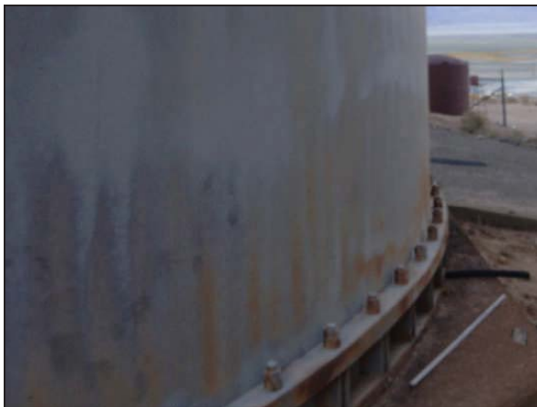
Picture 35—White metal exterior of the north silo.
