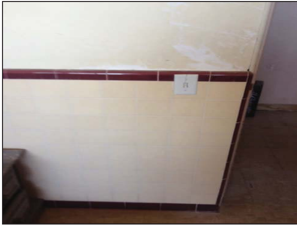
Picture 19—Red and beige ceramic wall tile found in the 2nd floor bathroom and room 4 in the house.
