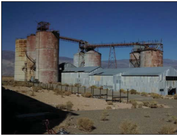
Picture 13—Mill and silos.
