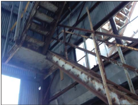
Picture 31—Gray metal staircase in the north end of the mill.
