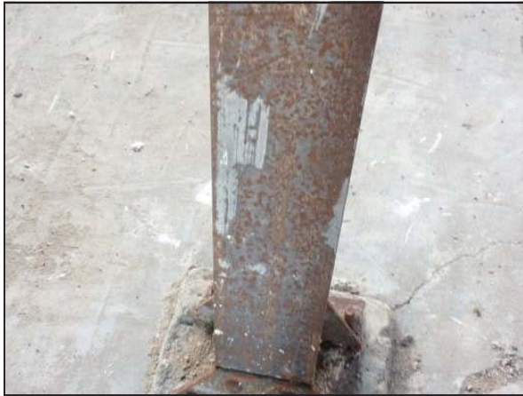
Picture 27—Gray metal hopper column found in the mill.
