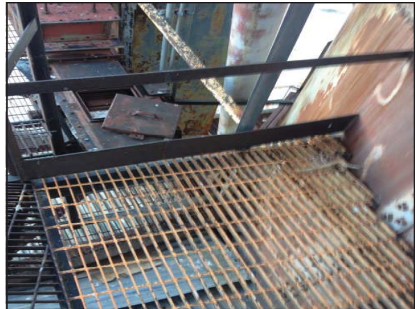
Picture 24—Orange grate on landing on exterior of east side of the mill.
