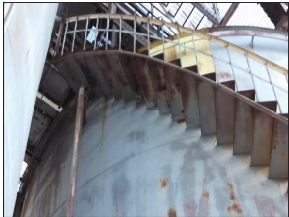
Picture 32—Gray metal staircase adjacent the north hopper, above the mill.
