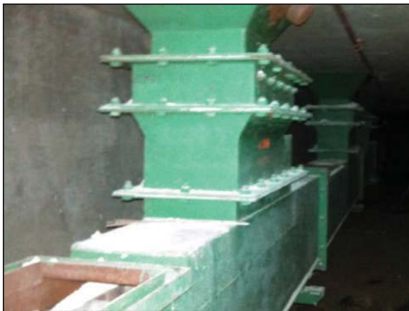
Picture 17—Hoppers in the basement beneath the silos.
