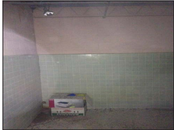
Picture 22—Green ceramic wall tile found in room 2 of the fabrication building.
