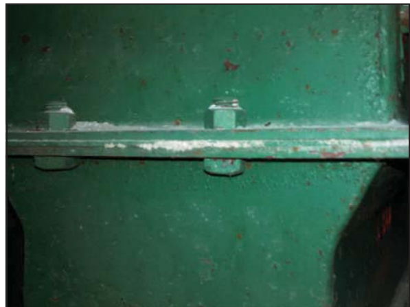
Picture 18—Gasket on the hopper beneath the silos.
