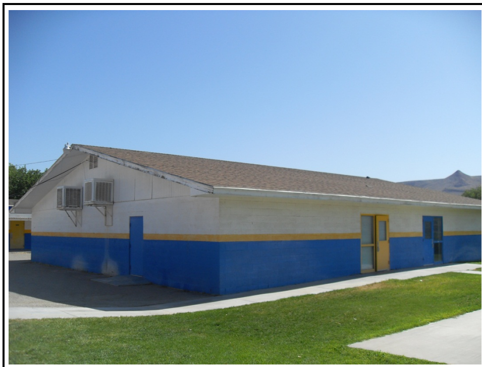
Photograph 8: Adjacent property to the east – school building
