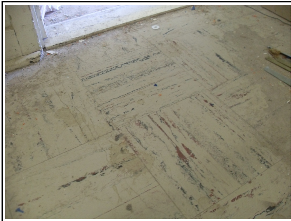
Photograph 17: View of tiles in maintenance storage room
