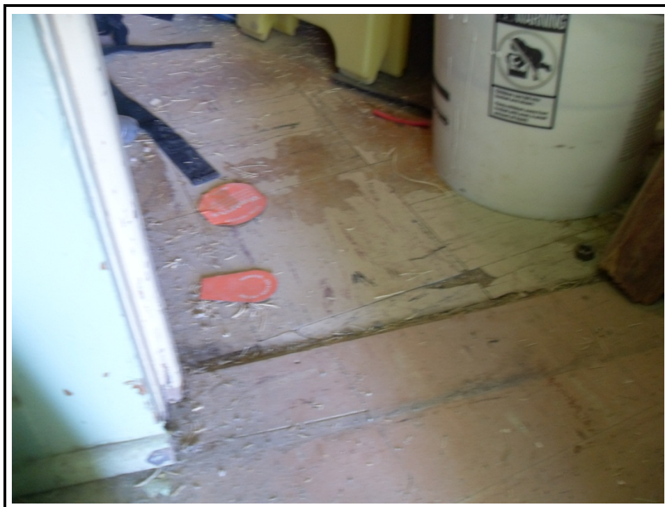
Photograph 18: View of various tile styles in maintenance storage room
