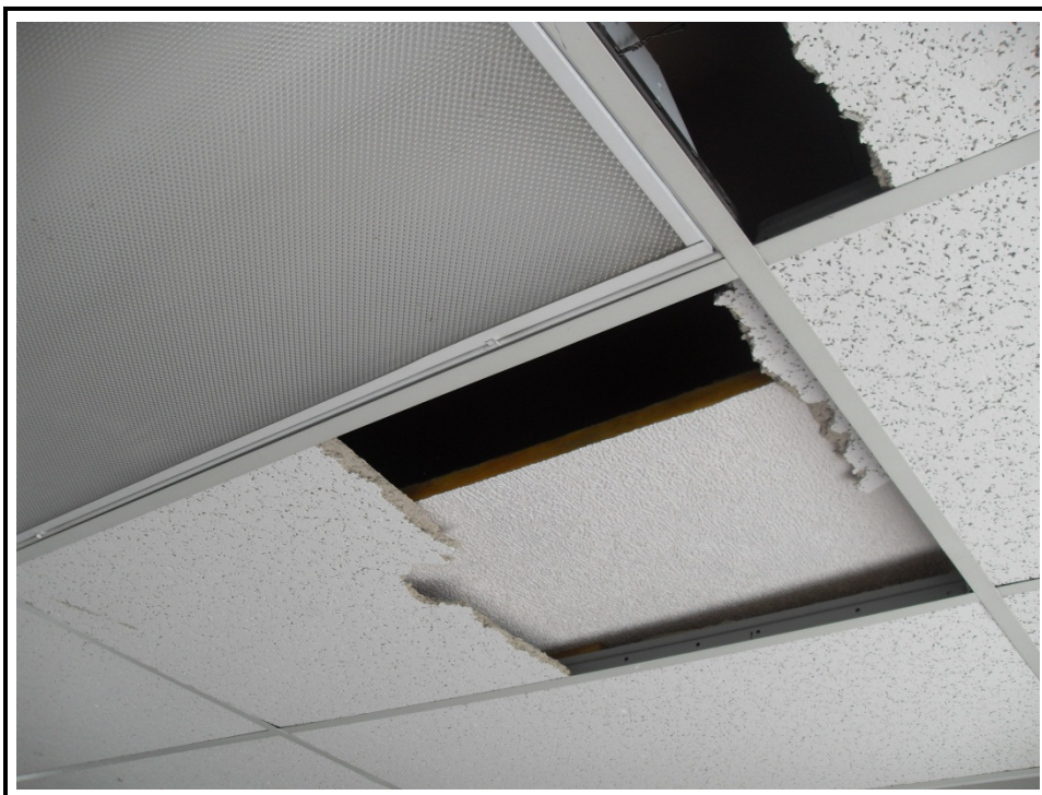
Photograph 14: View of insulated ceiling tile above drop down in weight room
