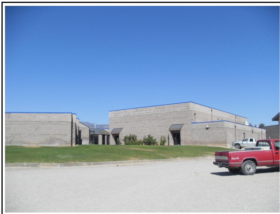
Photograph 10: Adjacent property to the west – high school facility
