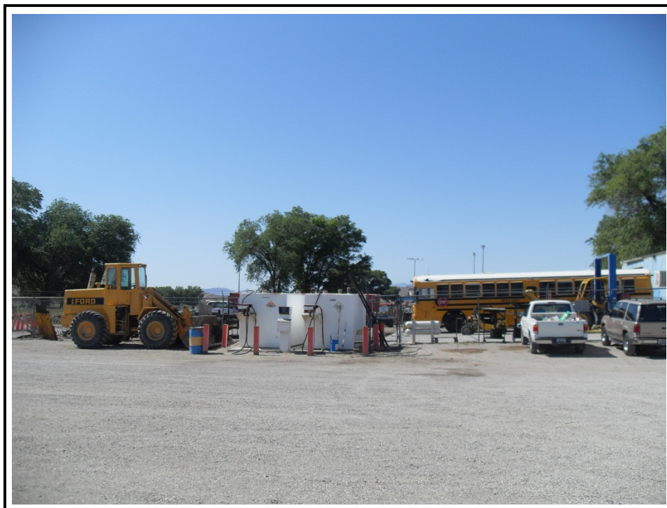
Photograph 24: View of above ground fuel tanks located to the south
