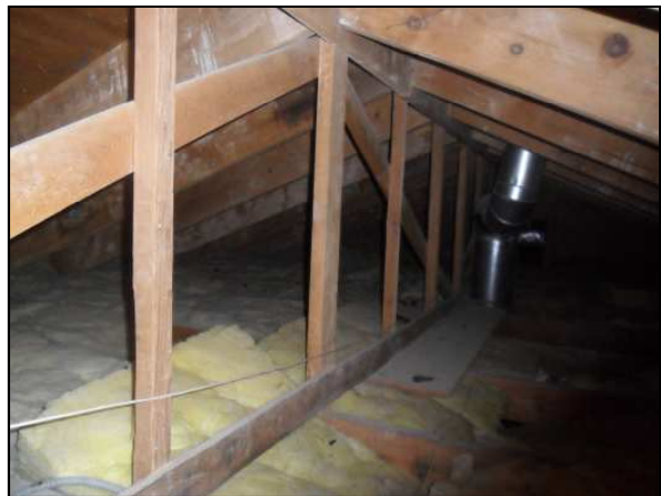
Picture 6 - View of Attic Space. No suspect ACM was observed.
