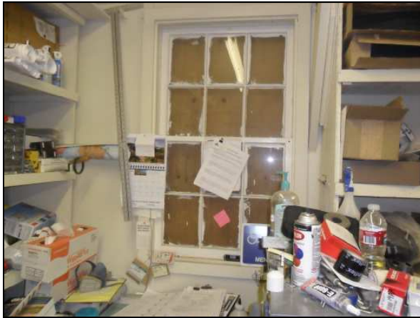
Picture 3 - Window Sash in the Maintenance Office.
