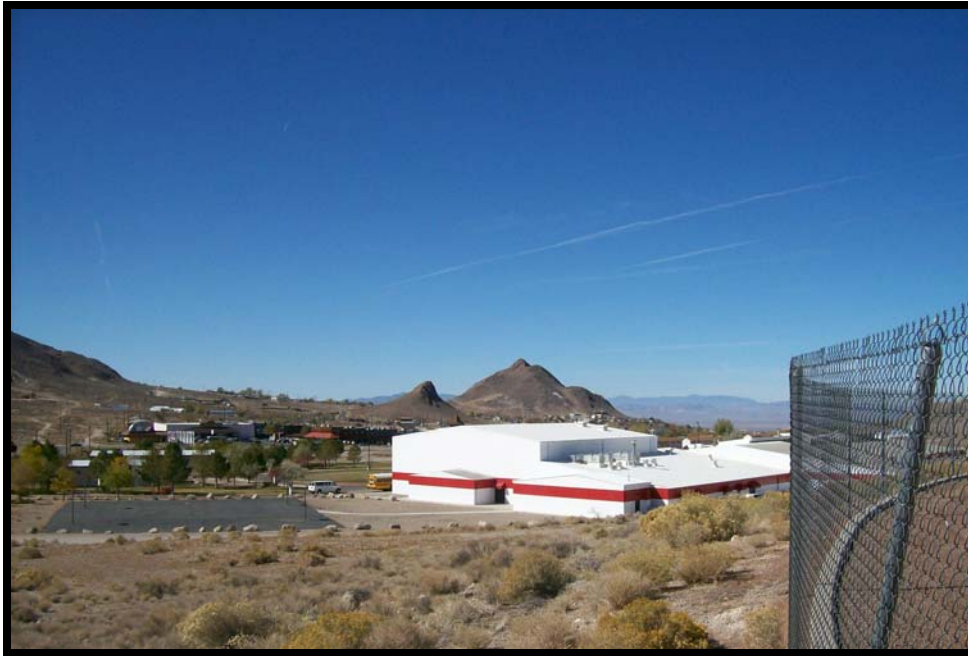
Photograph 3: View of Tonopah High School, facing northwest across Ray Tenant Lane.
