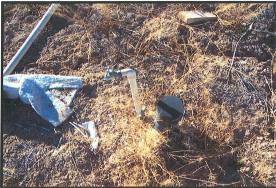
Photograph 14: View of septic system PVC pipe located on the subject site.
