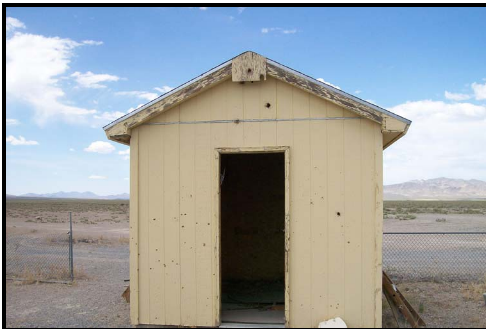
Photograph 10: View of former golf course storage building, facing north.
