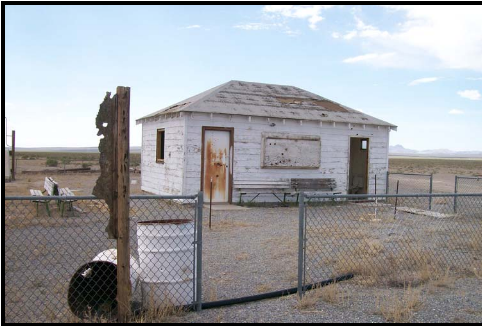
Photograph 1: View of golf course restroom building, facing northwest.
