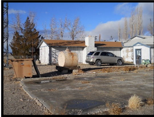
Photograph 5: Exterior of active FBO building and 1976 expansion, and view of fuel tank (looking north).
