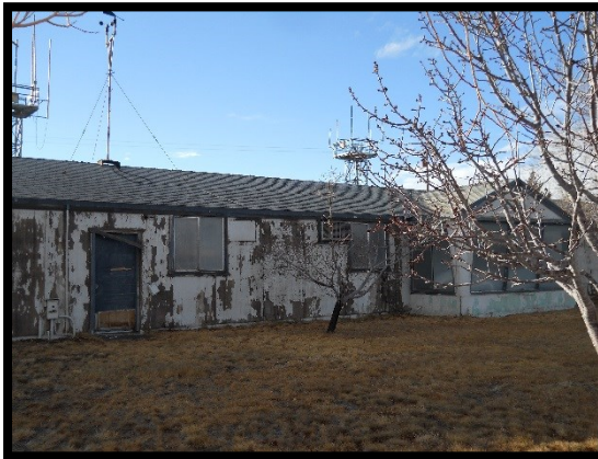
Photograph 3: Exterior of closed FBO building (looking west).
