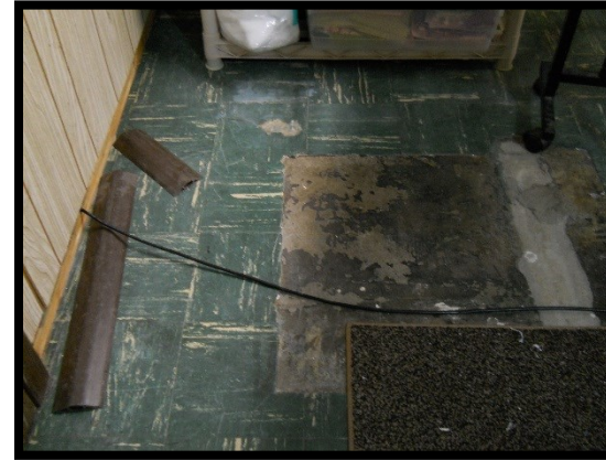
Photograph 12: Representative section of vinyl floor tiling and mastic in FBO building.
