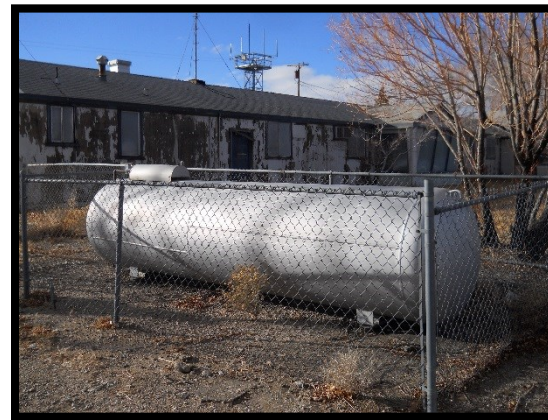
Photograph 8: Inactive propane tank at southeast corner of site (looking west).
