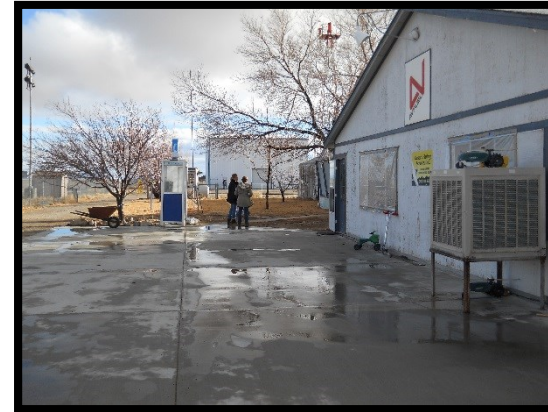
Photograph 2: Exterior of active FBO building and 1970s expansion (looking southwest).
