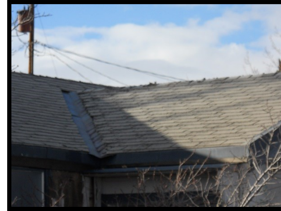
Photograph 6: Roof condition FBO building (looking west).
