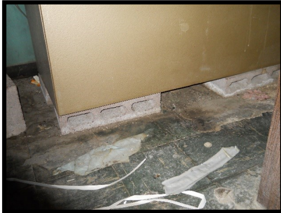
Photograph 11: Subsurface conditions under furnace.
