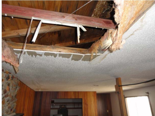
Acoustic Ceiling Spray 1976 Addition
