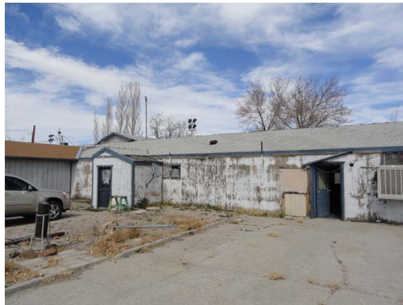
Exposed Pink And Green Paint Under Wood Siding Original Building
