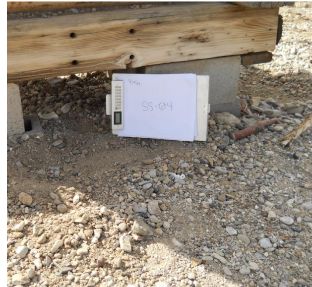
Photograph 6: Sample location of SS-04 at north end of tank
