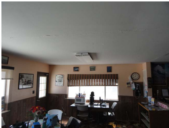
Textured Drywall (Ceilings and Walls) 1970 Addition
