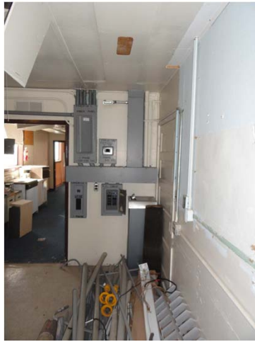
Transite Wall Paneling Looking North
