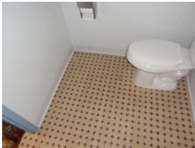
Ceramic Tile Over Remnant Sheet Flooring Bathrooms 1970 Addition
