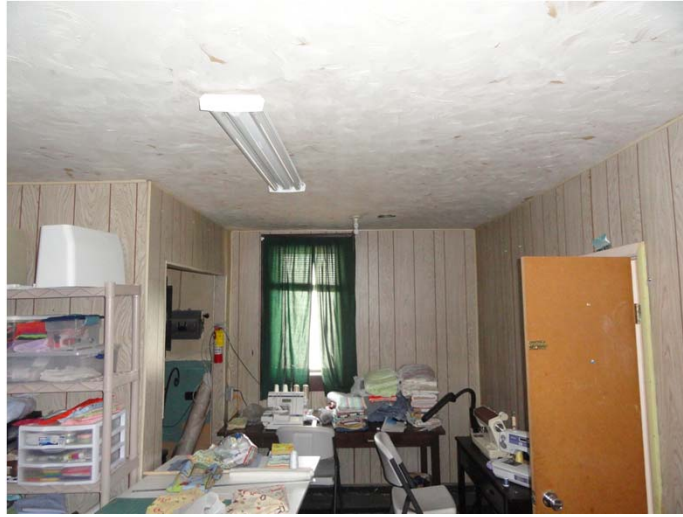
Acoustic Texture Sewing Room Original Building
