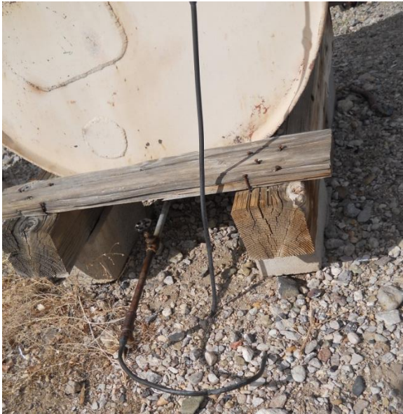
Photograph 1: West end of above ground storage tank
